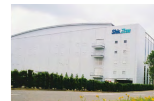
300mm wafer building (Shin-Etsu Handotai's Shirakawa Plant)
