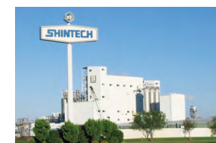
Shintech Freeport Plant (Texas, USA)
