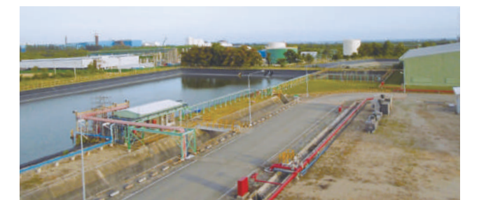
Rainwater is collected and used to provide industrial water to neighboring partner companies (Asia Silicones Monomer Limited)
