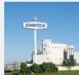
Shintech Freeport Plant (Texas, USA)
