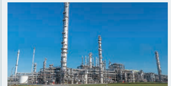
Shintech's ethylene plant that started operations in 2020 (Louisiana, USA)
