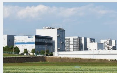
Yokonodaira Plant at the Gunma Complex (Gunma Prefecture, Japan), where capital investment to expand capacity is underway.
