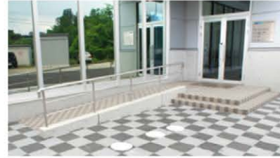
Wheelchair Ramps (Shin-Etsu Chemical Gunma Complex)
