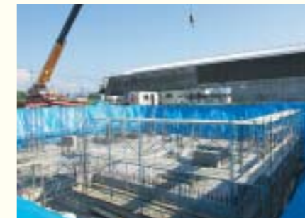
Expanded wastewater facilities under construction
