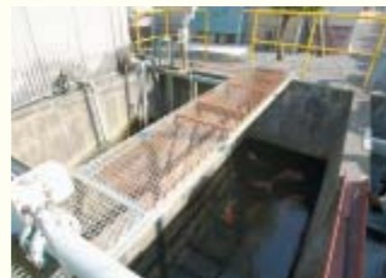
We keep carp at an in-plant pool that serves as the portal for release into rivers to help monitor wastewater in conjunction with instruments
