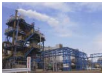
Raw material recycle facilities: Incineration (front, left) and recovery (back, right) facilities of the Naoetsu Plant's recycling system Shin-Etsu invested in and commenced full-fledged operation of an innovative new system that recovers emissions gas and salt water from wastewater, and reuses these as raw materials. (The incinerator's stack is giving off steam)
