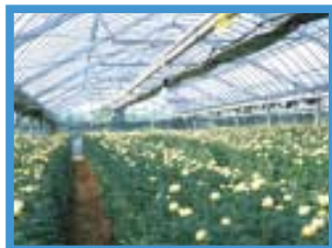
PVC sheeting is now widely used in greenhouses as an alternative to glass.
