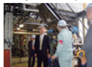
Special environment control and safety audit (conducted at JAPAN VAM & POVAL CO., LTD., in June 2007)
