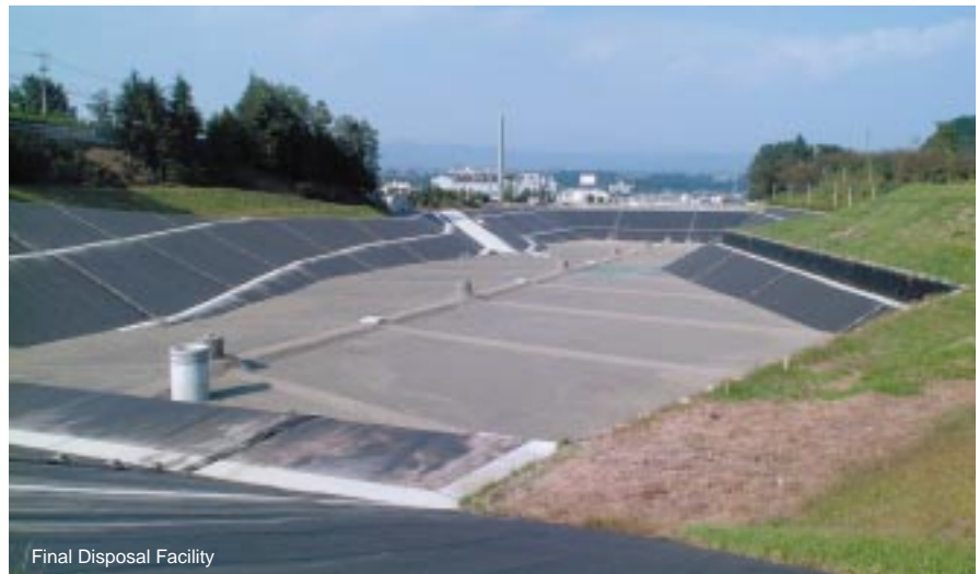
Final Disposal Facility
