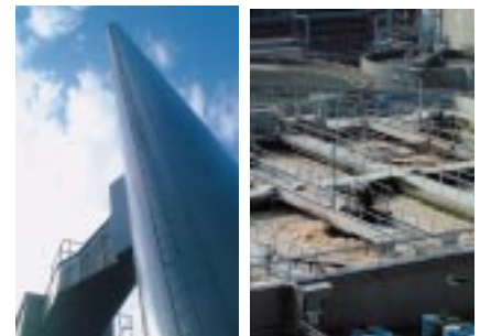
Left: The Co-generation System Right: The Waste Water Treatment Facility
