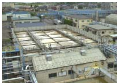
Water treatment facility
