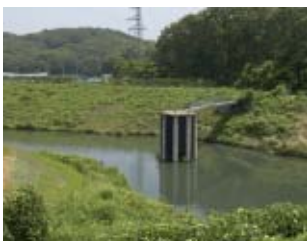
Water treatment facilities at the Shirakawa Plant
